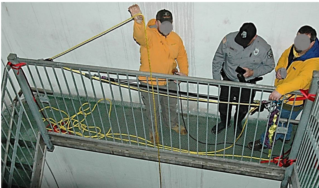
Figure 11- Haul system and lowering rigging post-accident.
